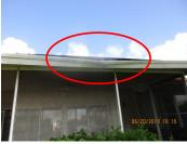
• **Repair:** The gutters require cleaning to avoid spilling roof runoff around the building – a potential source of water entry or water damage.
